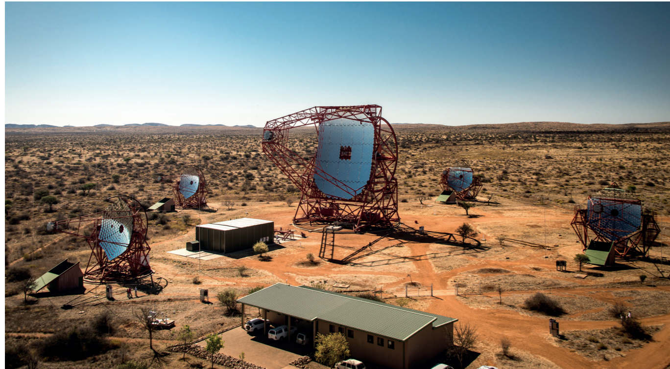
Fig. 2: The H.E.S.S. telescope system in Namibia, with the four 108 m 2 telescopes CT1-CT4 operational since late 2003, and the new 614 m 2 telescope CT5, inaugurated in 2012.
